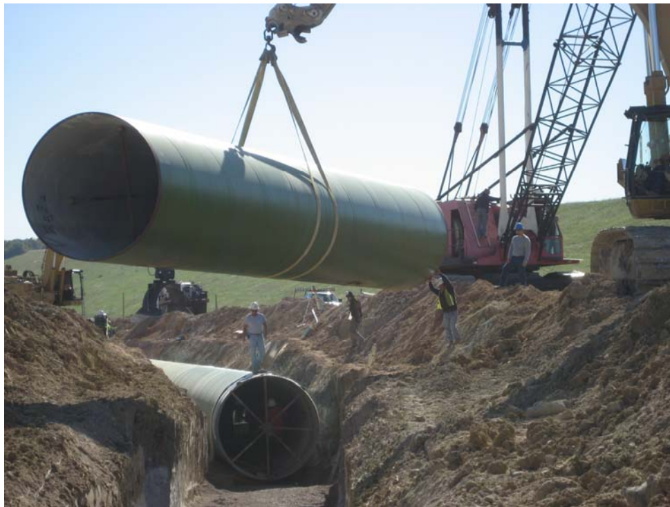
Figure 9. Eagle Mountain 96-Inch Polyurethane Coated Steel Pipe
