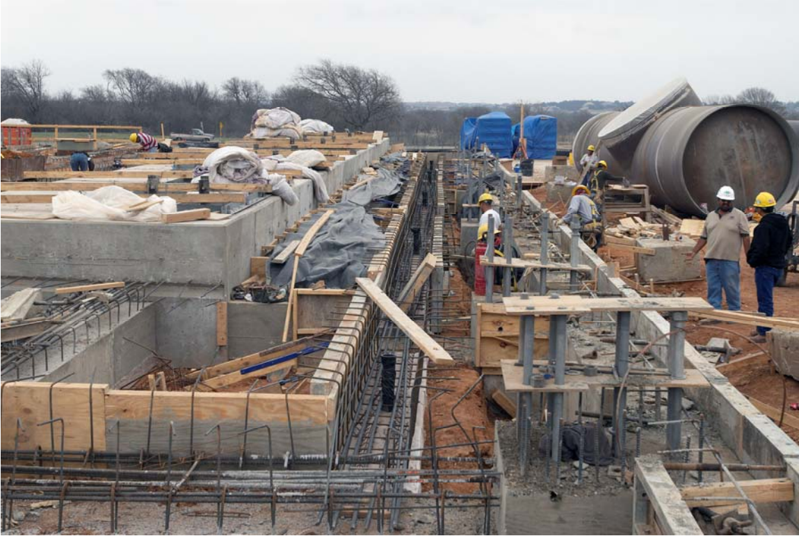
Figure 3. Benbrook Booster Pump Station Foundation
