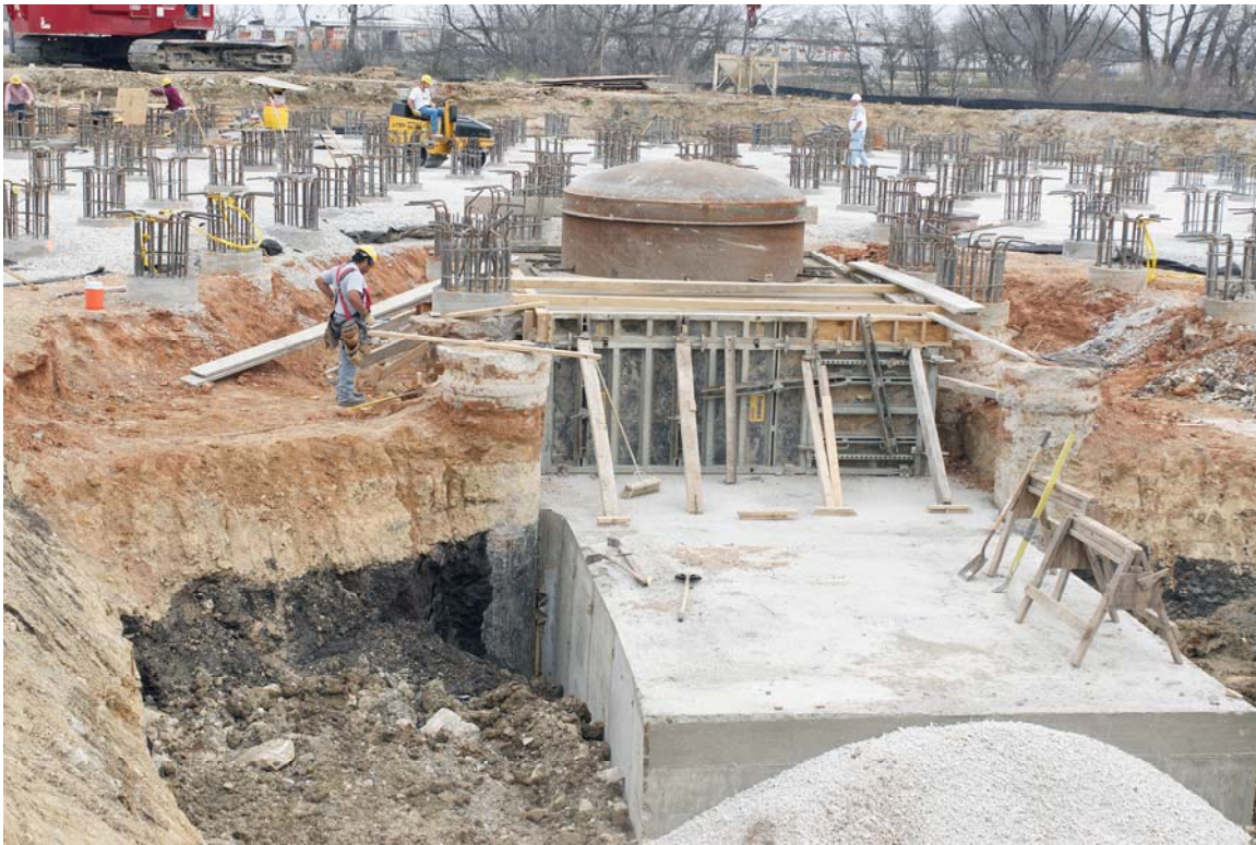
Figure 4. Drilling and Placing Piers for the Rolling Hills Tank Foundation
