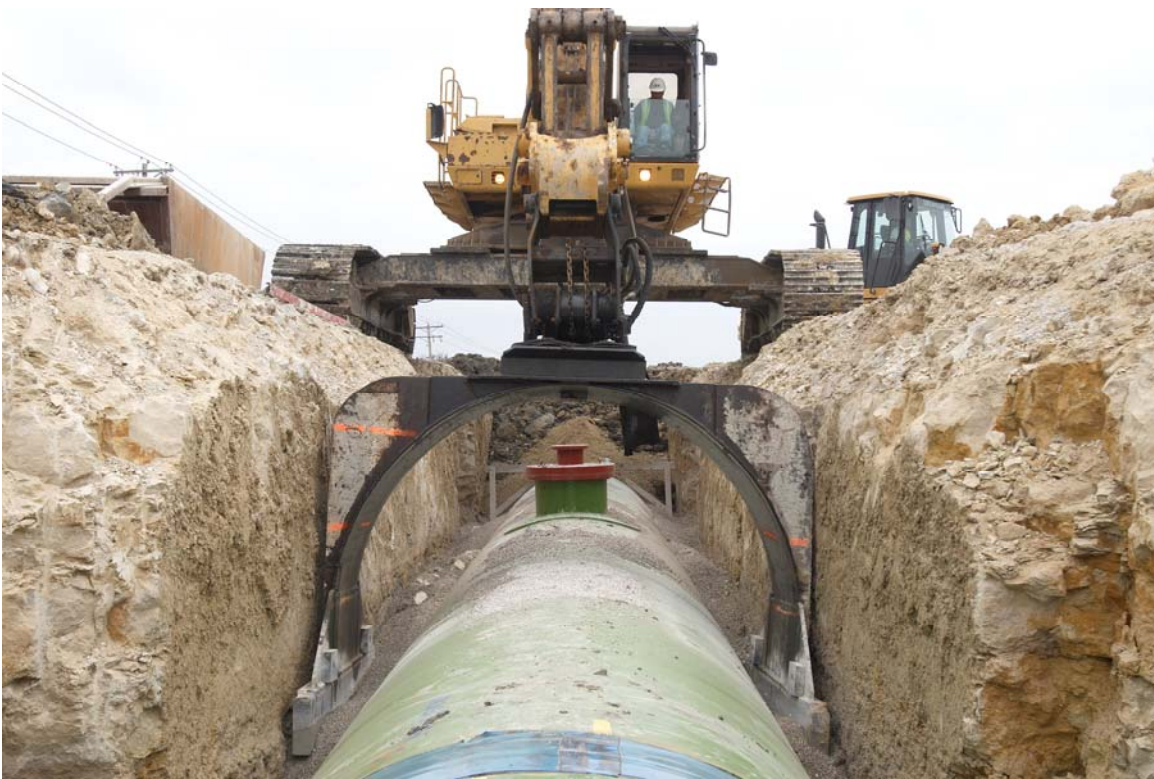
Figure 5. Vibratory plates for compaction of pipe embedment
