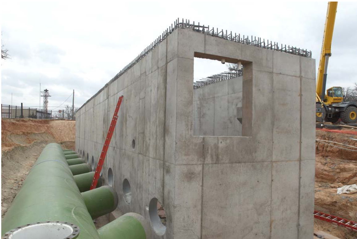
Figure 7. Construction of the Eagle Mountain Flow Control Vault
