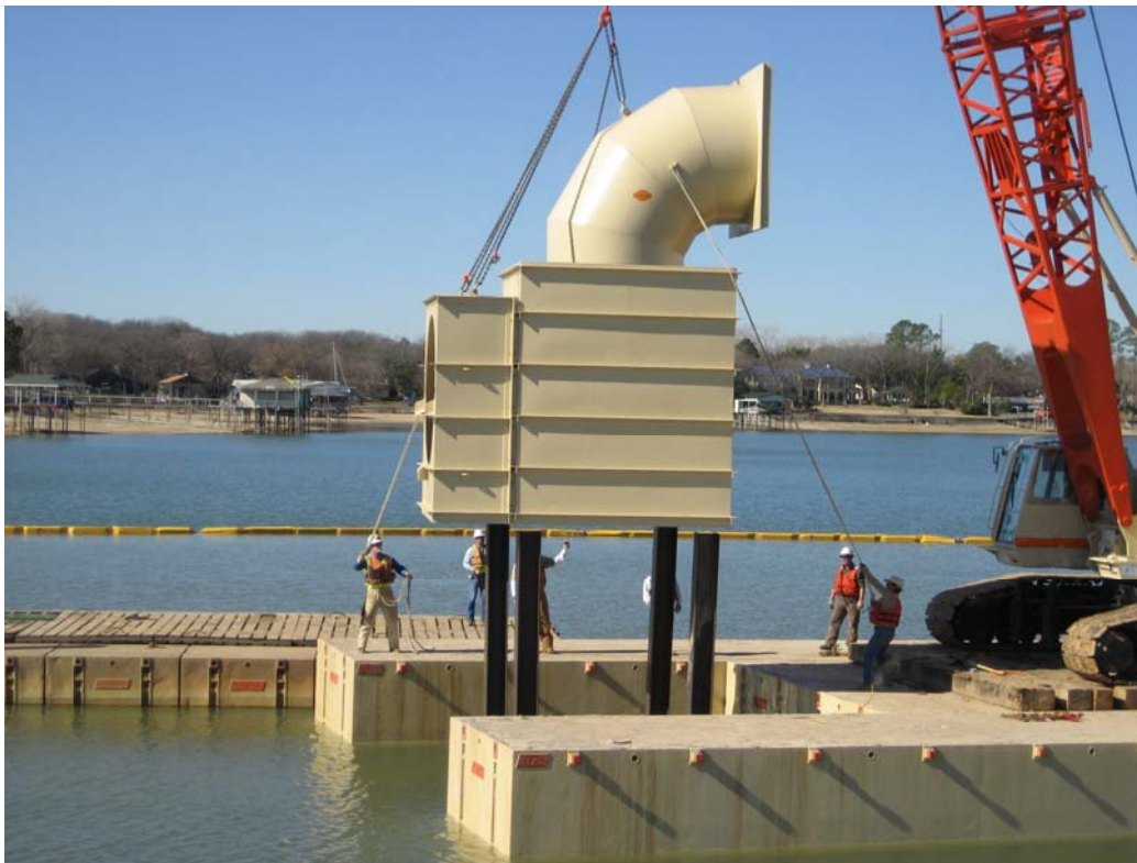
Figure 8. Outlet structure being positioned and lowered into Eagle Mountain Lake
