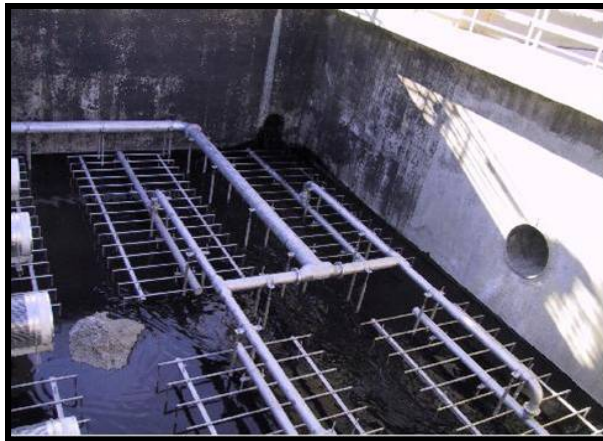
Figure 6 MBBR Diffused Aeration System
