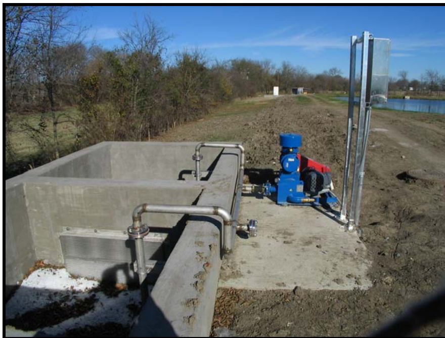
Figure 11 MBBR Structure Showing Reactor #1 Effluent Sieve White material in reactor is biocarriers (prior reactor going online)
