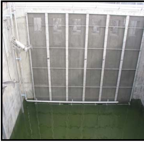
Figure 9 Typical Flat Screen Sieve Installations
