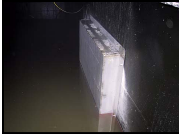
Figure 9 Typical Flat Screen Sieve Installations
