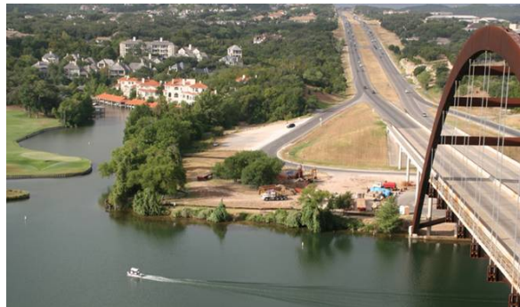
Figure 2 – Lake Austin and Penny Baker Bridge: The City and Austin Energy partnered to install new force mains and electrical conduits to serve the Davenport Ranch development near the picturesque Lake Austin and Penny Baker Bridge.
