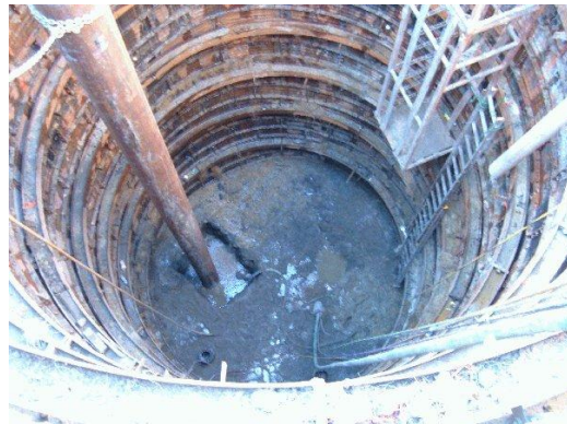
Photo 4. Intake vault shaft excavation
