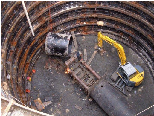
Photo 1. Sump excavation and suction pipe
