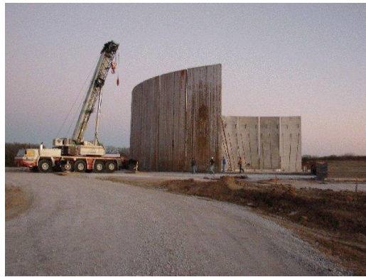
Photo 4. 6 MG tank wall construction
