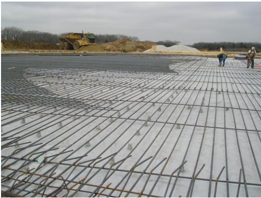
Photo 3. 6 MG tank foundation reinforcing
