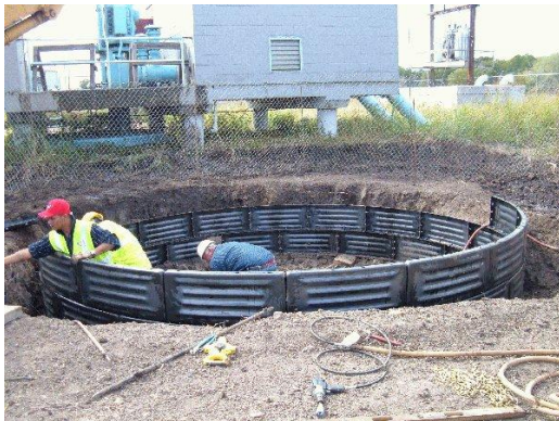
Photo 3. Intake vault liner plate at surface
