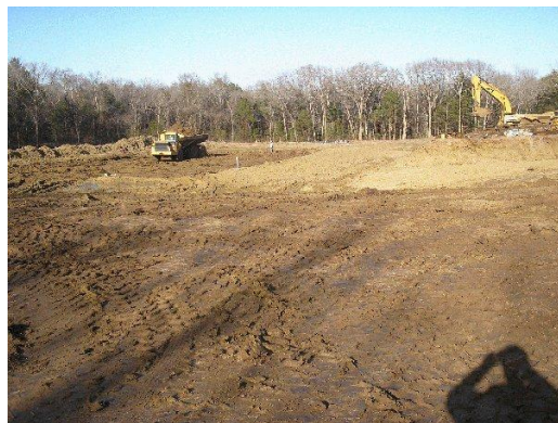
Photo 6. Intermediate PS excavation
