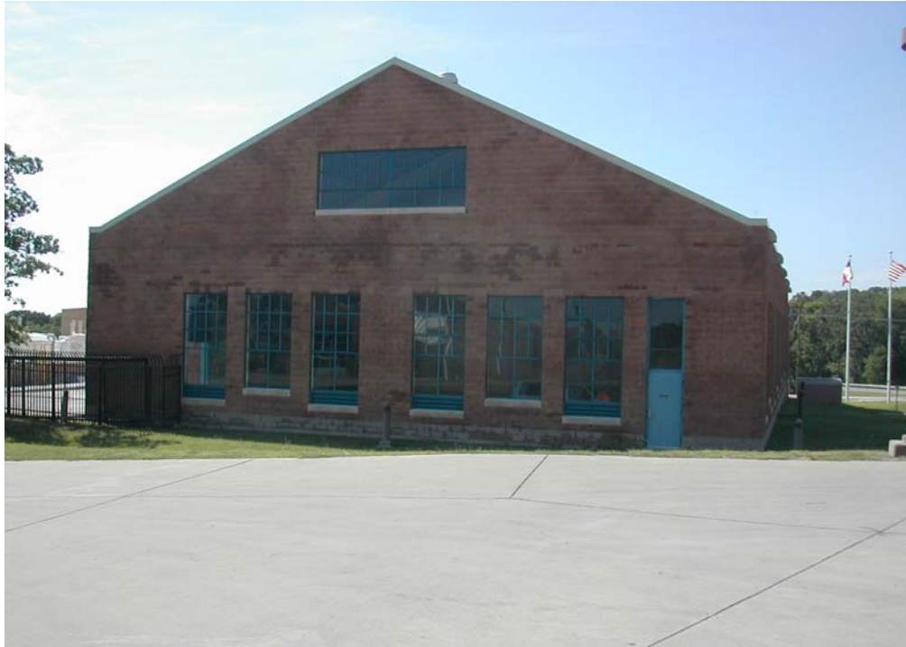
Figure 2 – Weatherford Water Purification Plant Treatment Building
