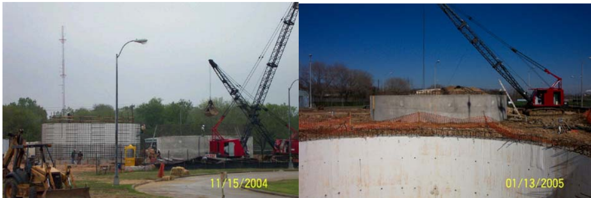
Figure 3: New Caisson Influent Lift Stations Construction
