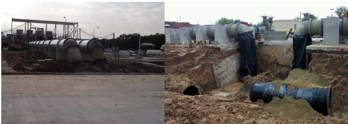
Figure 4: New Influent LS Force Main Construction
